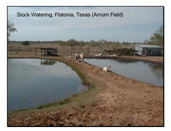
Another photo from Flatonia. The pond on the right has some floating oil (note the black rim around the edge). This is retained and the skimmed water is routed via a subsurface pipe to the pond on the left. The production well is just off the photo to the right.
