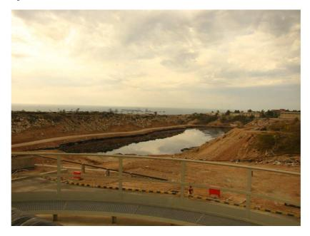
Figure 1. Retention pond for oil-water separation, Kharg Island, Persian Gulf, South of Iran
